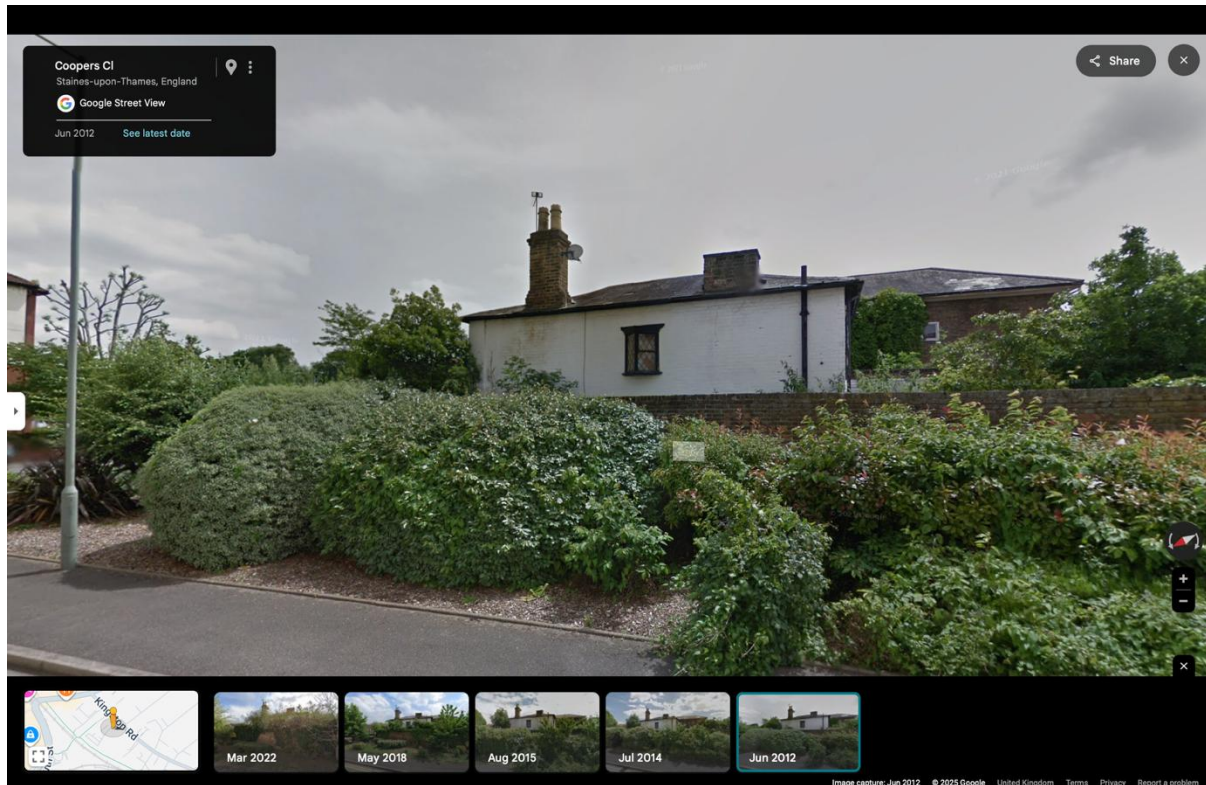
Photo 2- West Elevation – Site in June 2012 - Copyright Google Maps.
