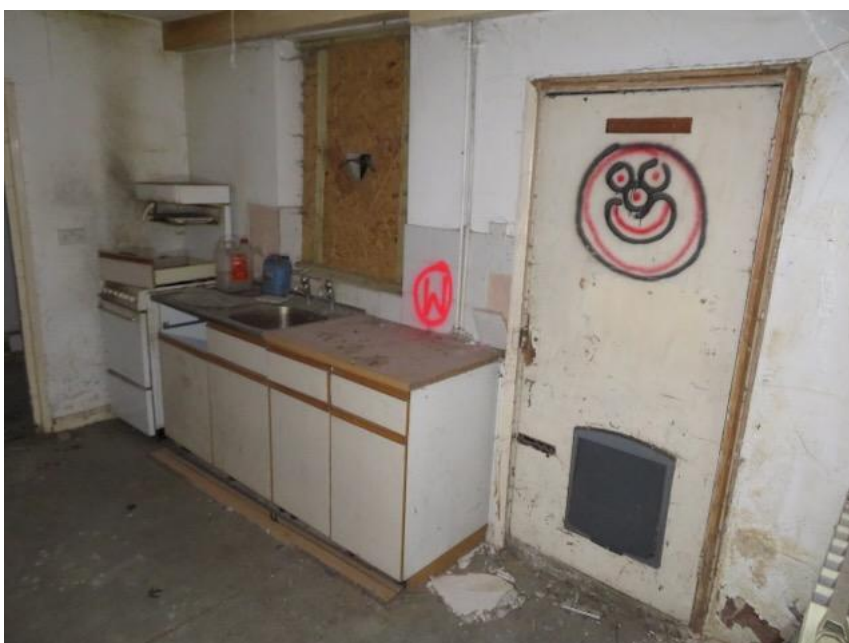
Photo 13- Guano covered derelict kitchen
